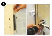
Lock and handle suitable for the leaf are fitted by screwing them.
