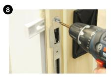
Lock is screwed to the drilled area in the frame.
