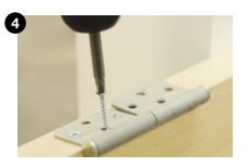
Hinges are screwed to the leaf with the upper hinge center 250 mm and lower hinge center 300 mm.
