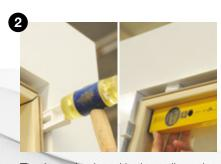
The frame is placed in the wall gap in the middle. Squeezing pins are placed in the upper and side gaps and fixed by adjusting with the measurement gauge.
