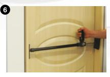
Adjust the internal measurement between sashe and frame as 3.5 mm by using an adjuster. Frame - Sashe balance should be checked again.
