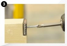
For Deodara range doors, ADOKAPI label is screwed on the lower and upper edge of the leaf as shown in the figure.
