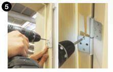
Upper hinge center is screwed to the frame as 254 mm from above.
