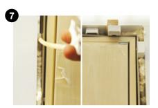
Apply polyurethane foam in the gap between the frame and wall. After drying, remove the foam residues.
