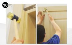
Double-side adjusted cornice are cut according to the measurement and fitted by using a plastic hammer.
